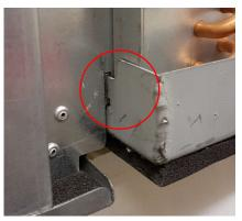
Fig 8.2b: Drain Tray Rear Support Lugs
