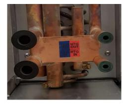
Figure: 5.4a Identification of heat exchanger coil connections
