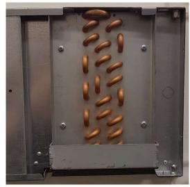
Fig 8.3b: Coil fixing screws
